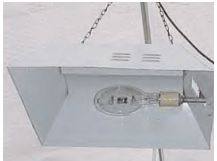
High Intensity Discharge light fixture.
